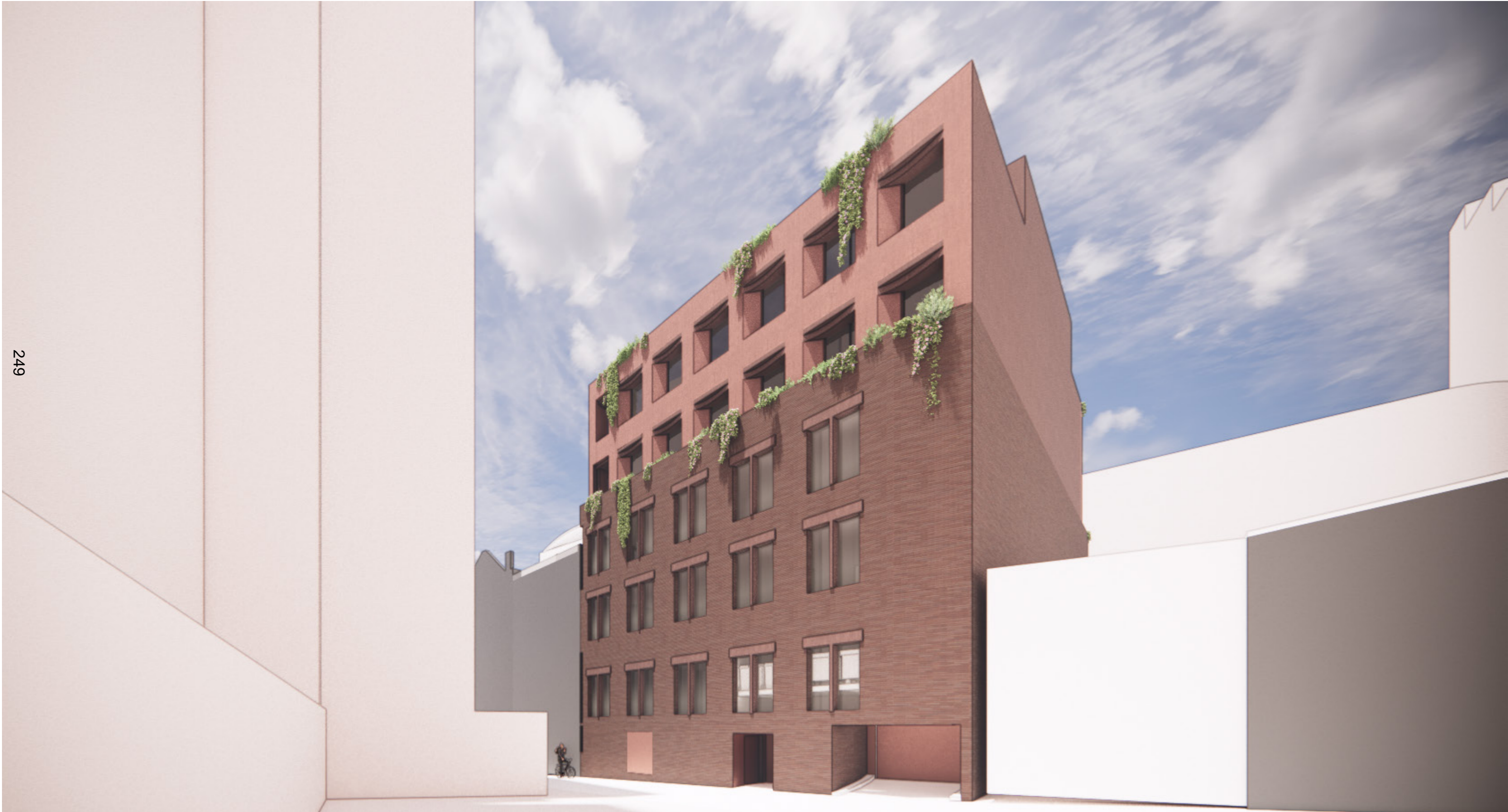
Busby Lane, looking at western elevation
